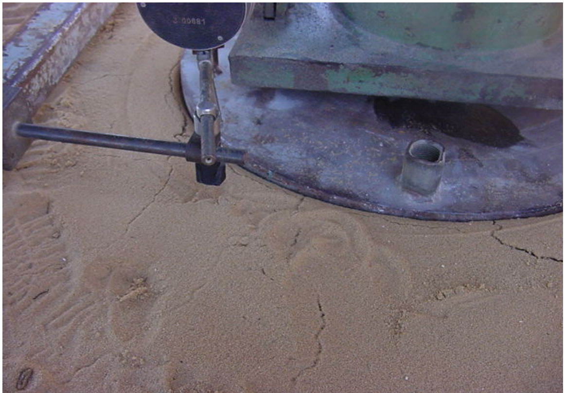
Figure C.4: A close up picture of the failure occurred in the sandy soil on site
