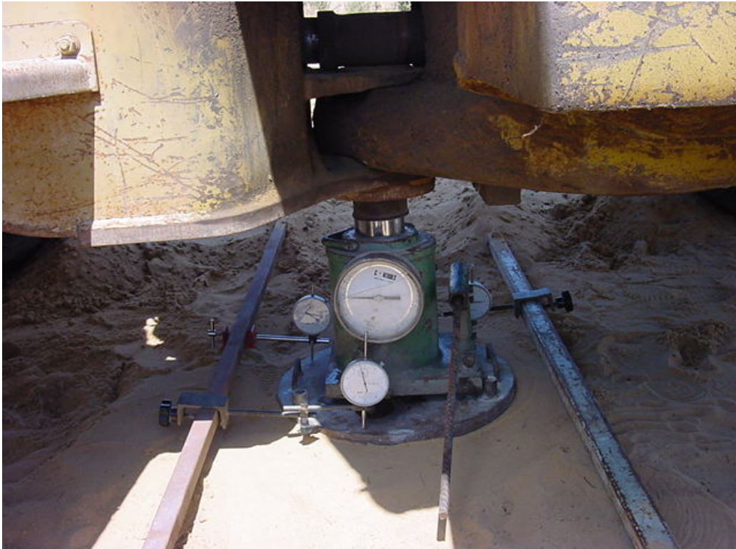
Figure C.1: A photo shows plate load set up and instrumentations
