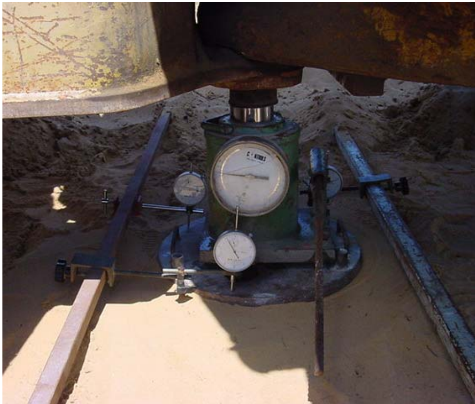
Figure (4.1): Arrangement for plate load test set-up
